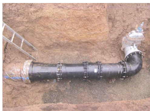
(導水管布設工)
